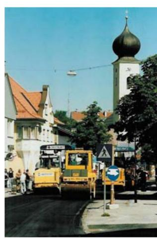
Road-laying at reduced temperatures at Fernpass
