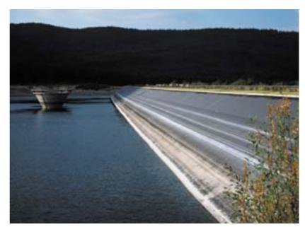
Drinking water dam – sealed with asphalt
